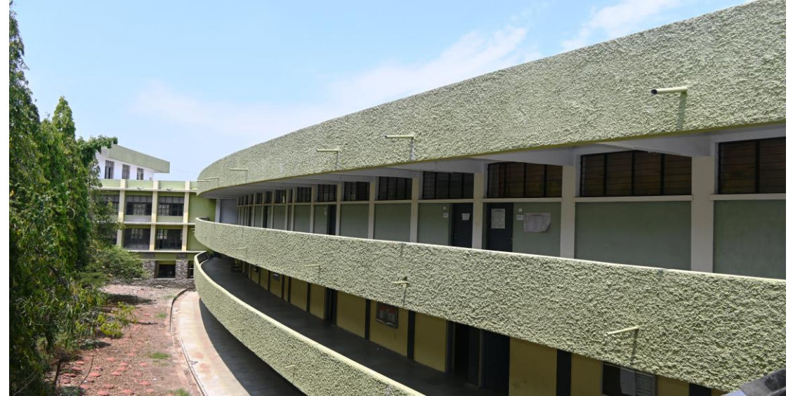
Construction of 6 new classrooms
