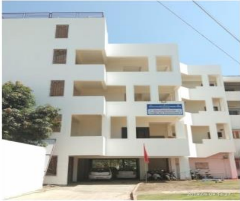
New Construction : 4 classroom
