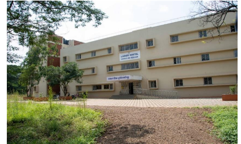
New Construction of Girls Hostel
