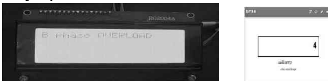
Figure 14: overload fault detection of B phase.
