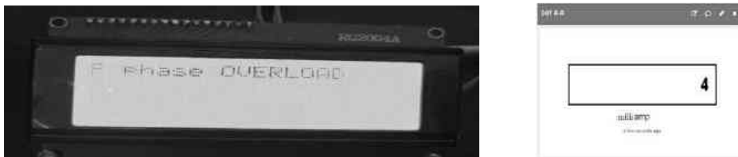
Figure 12: overload fault detection of R phase
